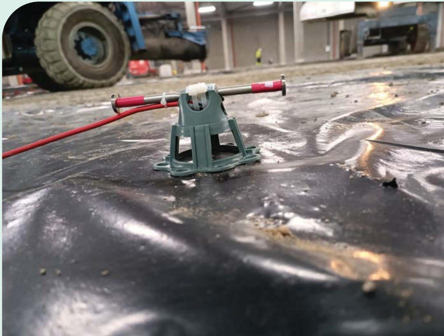
LEFT: Figure 6 – installation of VWSG sensors at Primekss jobsite.
